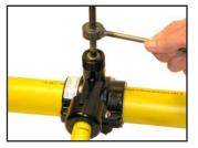
Tighten the compression nut until it shoulders against the outlet. Do not overtighten. **CAUTION:** To prevent inadvertent pull-out of the P.E. tubing during the assembly process, complete step 11 immediately after step 10, without delay and ensure work is not being performed on the free end of the P.E. tubing.
