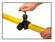
together along the outer edge. The flanges of the saddle may not come together next to the pipe. Bolt torque should not exceed 120 inch pounds.
