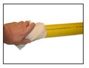
8 Mark the stab depth on pipe. (See below. Stab Depth Lengths are to scale and may be used to measure stab depth.)
